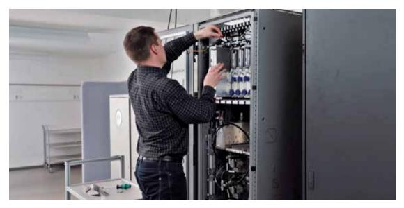
5. The switch which distributes the backhaul to both the eNodeB and TETRA radios is installed just below the eNodeB.
